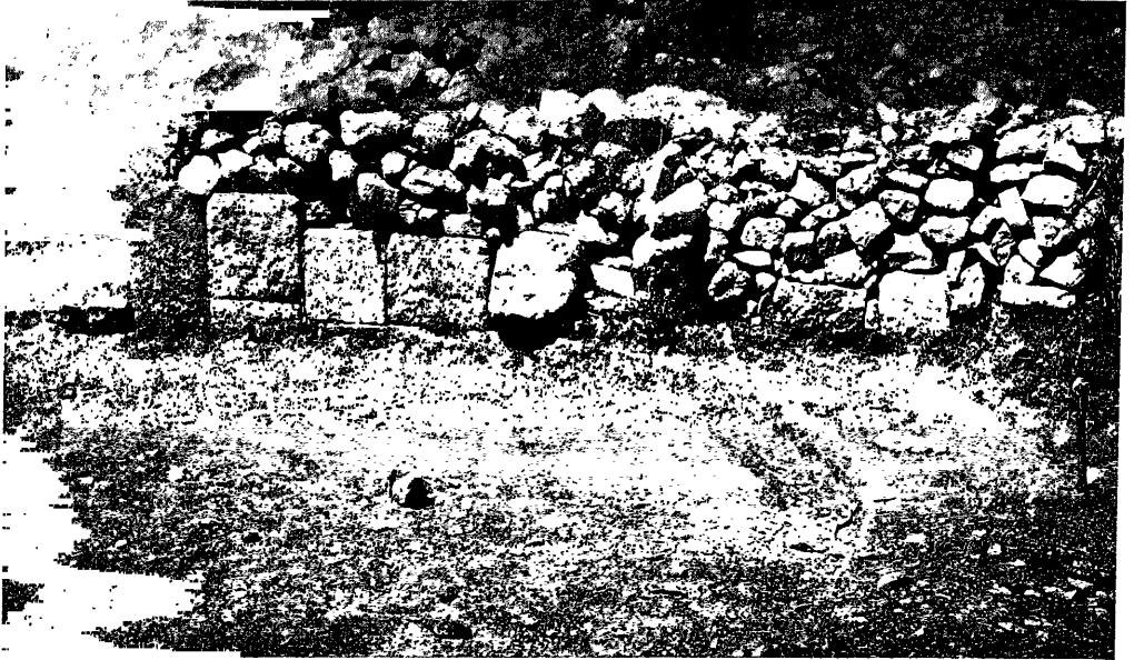
FIG. 1. SUHMĀTĀ CHURCH: APSE, LOOKING NORTH
